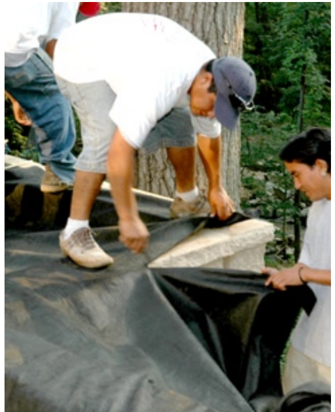
Installing the Geotextiles (optional)
