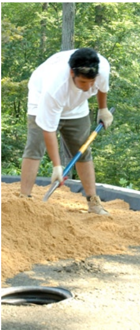
Installing and Leveling the Bedding Sand
