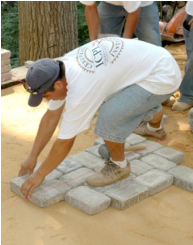
Installing the 1st pavers
