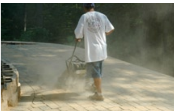
top left: Pavers compacted in place before spreading of joint sand. middle left: Spreading and sweeping of joint sand. bottom left: Compacting with joint sand. right: The finished patio.
