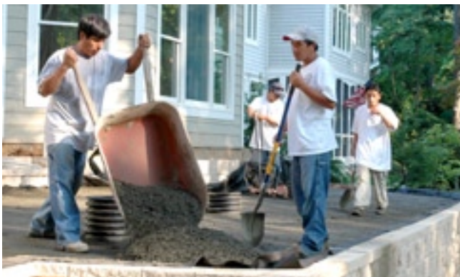
Installing the Base Aggregates
